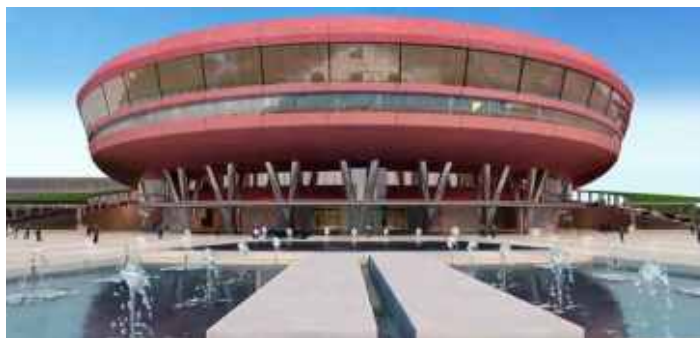
Ongoing Project of I.T.P.O. Convention Centre Building at Pragati Maidan, New Delhi
